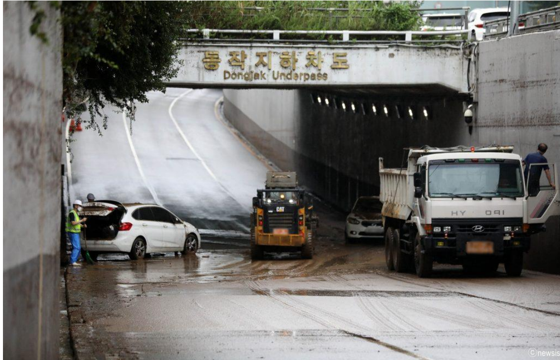
Flood damage in Seoul, South Korea, August 2022. Photo: Government of Seoul
